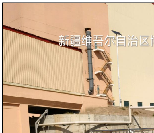
垃圾坑非正常工况排气筒
